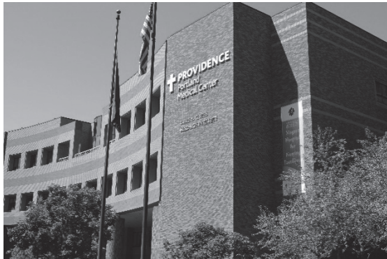
写真2 Portland Providence Medical Center
